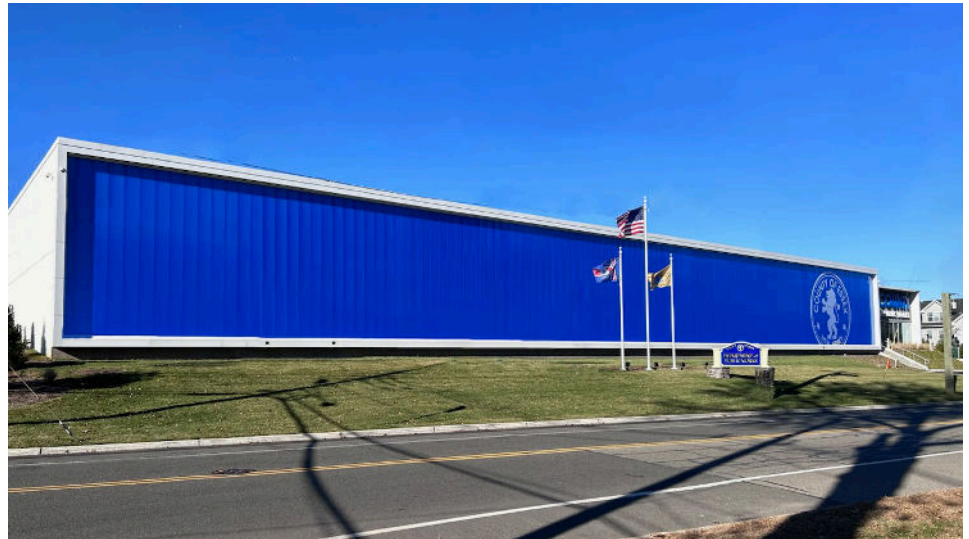
Essex Co. Public Works building features blue ThermaLite Plus
